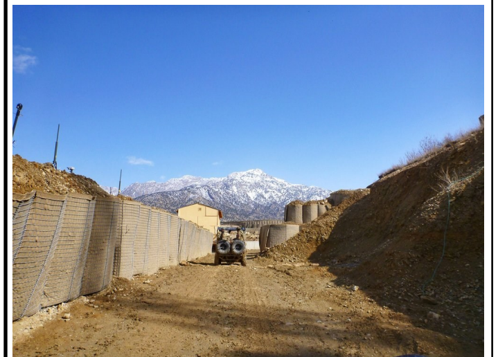
HESCO walls lining the Combat Outpost in eastern Afghanistan. Courtesy of Jackie Munn
